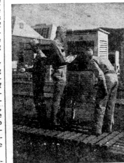
Here the men are obtaining temperature and humidity readings. The man on the left is whirling a sling psychrometer in order to determine the relative humidity and dew point.
