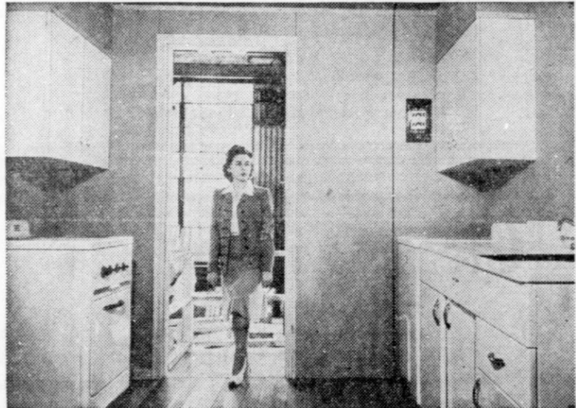
Everything but pork chops! A few hours after the first section of the "demountable" was put in place, milady enters the kitchen and finds it completely equipped and ready for business.
