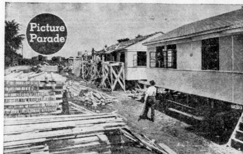
On the assembly line at Muscle Shoals, Ala. The houses being built here are made in uniform-sized, portable sections, and can be put together in about four hours.
