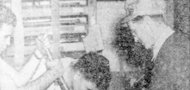
Working, forging, woodworking, operation and repair of motors are courses being offered. Above, students learn how to cut the Schenley company's machine shop at Frankfort, Ky., where they were taken. Plant technicians donate their services as
