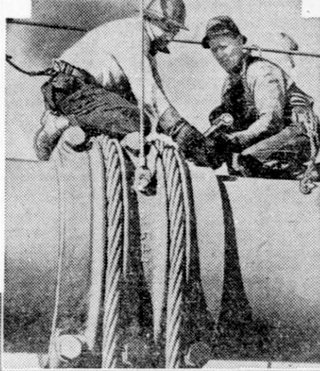
Above: Twenty experienced painters working daily daub 8,000 gallons of paint annually on 100,000 tons of structural steel and 80,000 miles of tough wire cables in an effort to prevent deterioration of the world's tallest and longest single span suspension bridge. Right: Seven hundred forty-six feet above Golden Gate, two men inspect main "saddles" and weatherproof shrouds of the 36 1/2 inch diameter steel cables.
