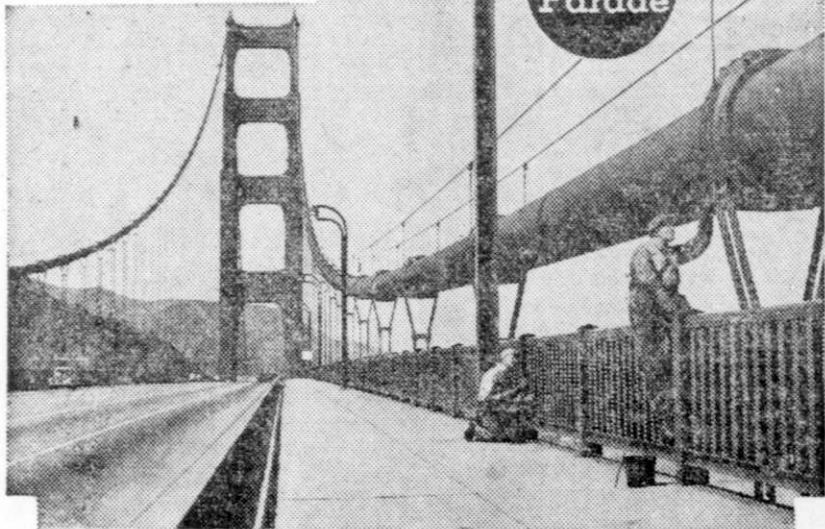
Above: Twenty experienced painters working daily daub 8,000 gallons of paint annually on 100,000 tons of structural steel and 80,000 miles of tough wire cables in an effort to prevent deterioration of the world's tallest and longest single span suspension bridge. Right: Seven hundred forty-six feet above Golden Gate, two men inspect main "saddles" and weatherproof shrouds of the 36 1/2 inch diameter steel cables.
