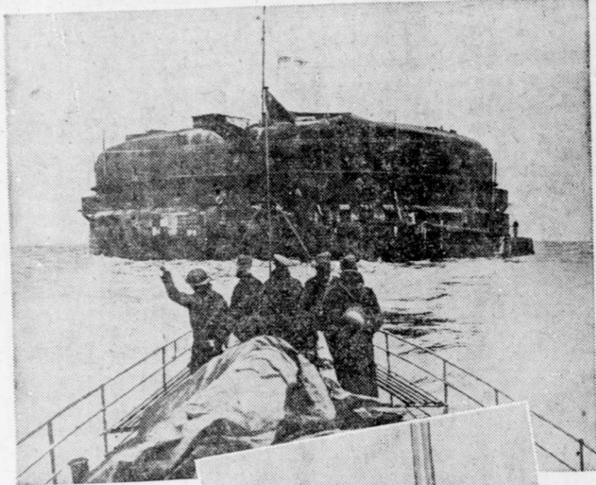
Above: Approaching one of Great Britain's formidable forts of the sea. These giant masses of steel and concrete, literally bristling with guns, are a new departure for war, and so far as England is concerned, a good investment. They are planted in "strategic" spots around England.
