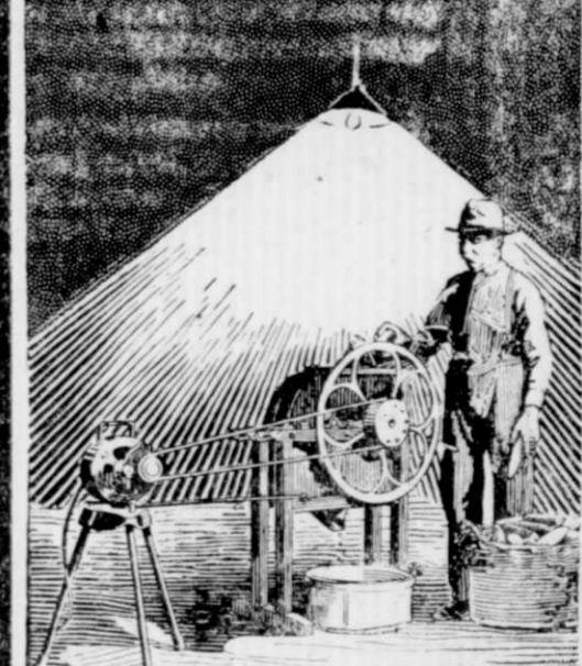
PUMPS the WATER
