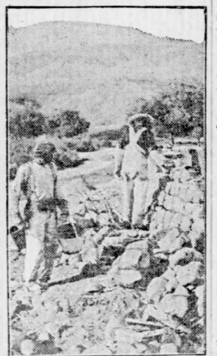
Construction of Cobblestone Masonry Wall.
