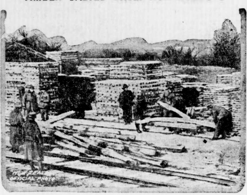
Salvage is playing a great part in the present war. This photograph shows timber salvaged from German dugouts that has been cut up in the sawmills of the New Zealand Tunneling company to be used in the construction of dugouts for the troops.
