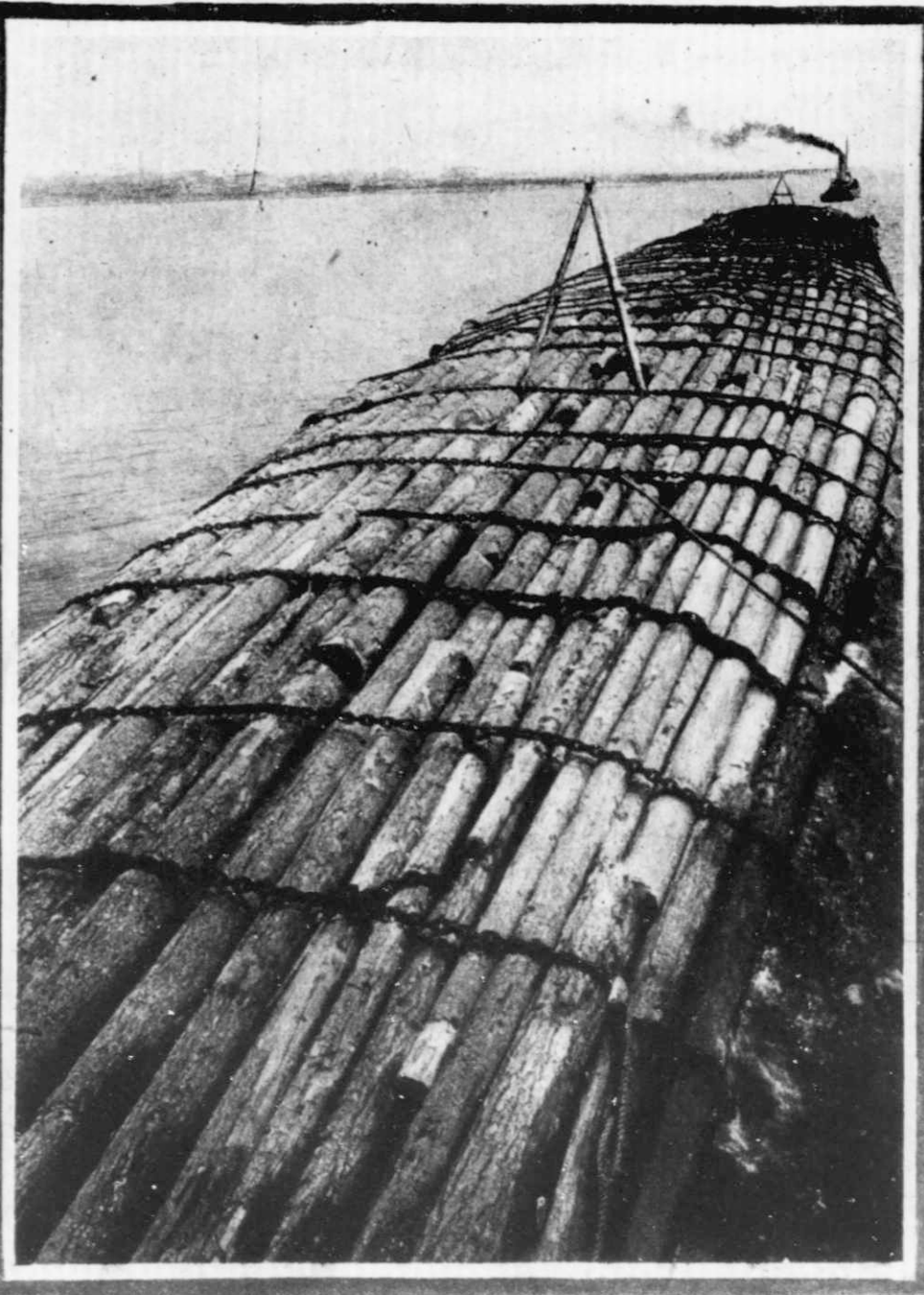
Army Lumber Is Sent South in Huge Log Rafts. Oregon Pine Logs Sent from a Point on the Columbia River, Oregon, 1000 Miles from Its Mouth, Floated Down the Pacific Coast from San Pedro to San Diego. The Lumber Structures, for Such They Are, Measure 800 Feet in Length and 52 Feet in Width, and the Current Shipment Totals 8,000,000 Feet of Sturdy Logs. Each Log Is 80 to 100 Feet Long and About Four Feet in Diameter.
