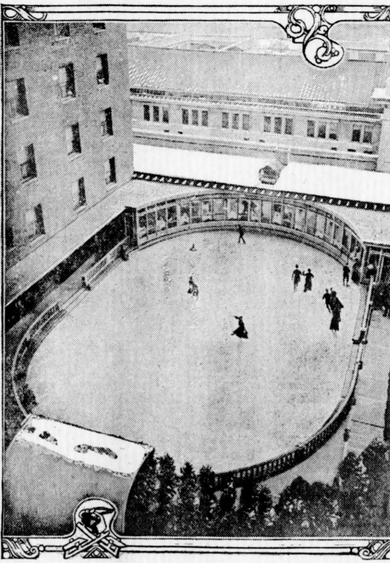
An enterprising New York hotel has laid out an ice skating rink on its roof. Inclosed tea rooms circle the rink.
