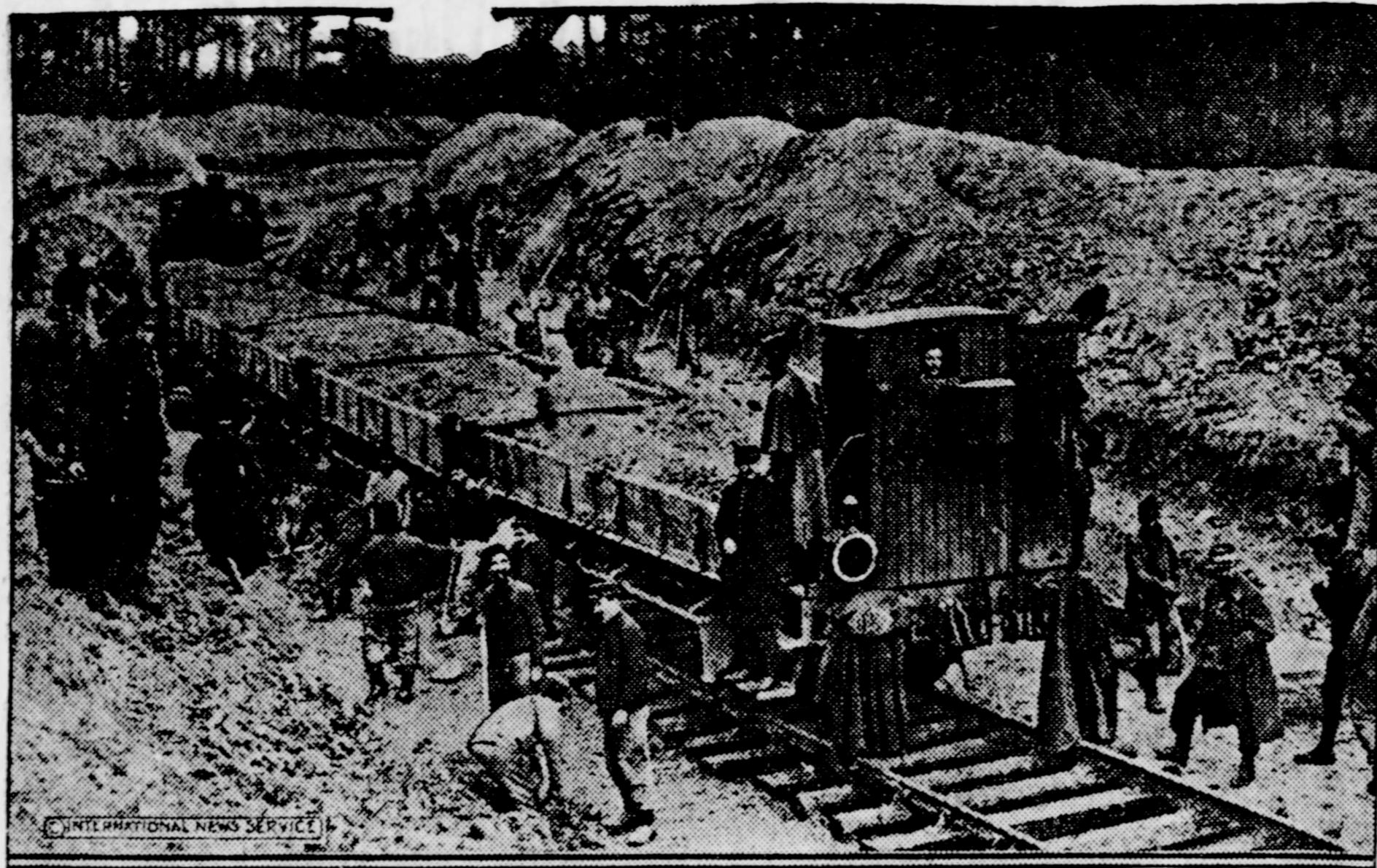
In three weeks the French engineering corps completed a one-track railway line running from Versailles to Compiègne so that troops can be transported to the front without passing through Paris. The road runs through the woods of Empress Josephine's Malmaison estate.
