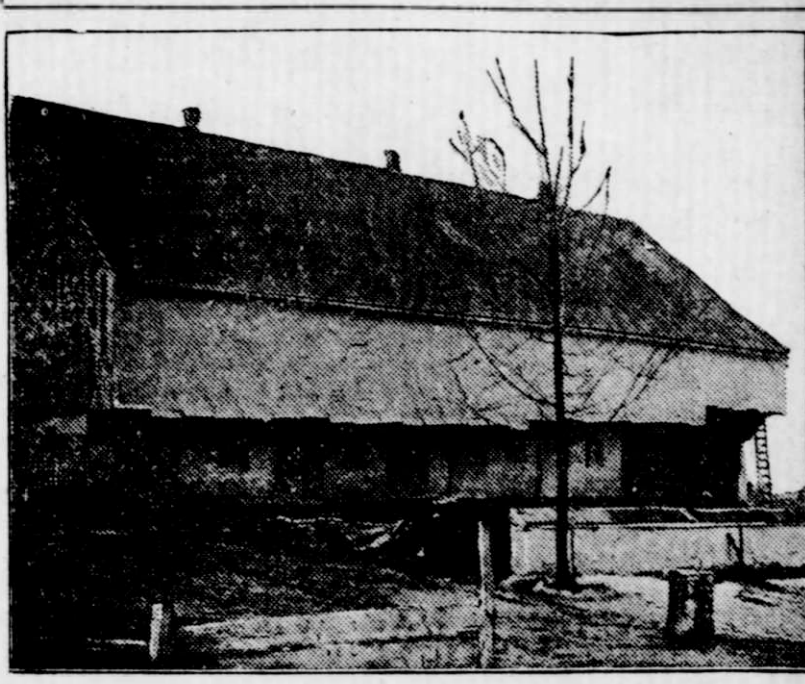
Building Prepared for Disinfection—In This Case the Disinfecting Was Done by Fumigation—Openings in the Barn Were Closed by Paper to Prevent the Escape of the Gas.
