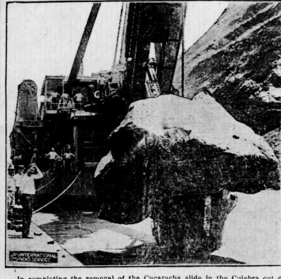
In completing the removal of the Cucaracha slide in the Culebra cut of the Panama canal this powerful new dredge, Bucyrus, is being employed. It is here shown picking up a 40-ton boulder.
