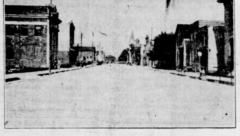
Street as it Appeared After Completion
