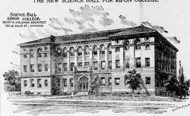
The material used in the construction of Science hall, Ripon college, is vitrified, dark-red brick with trimmings of Bedford stone, and the style of architecture is classic. In size the building is 181 x73 feet, and, including the basement, four stories in height. On account of the slope of the hill the basement on the south side through a fine doorway.
